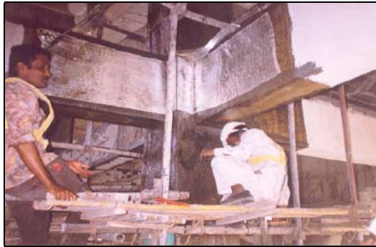
Photo 6 : Application of Slide Wrap on beam column junction
