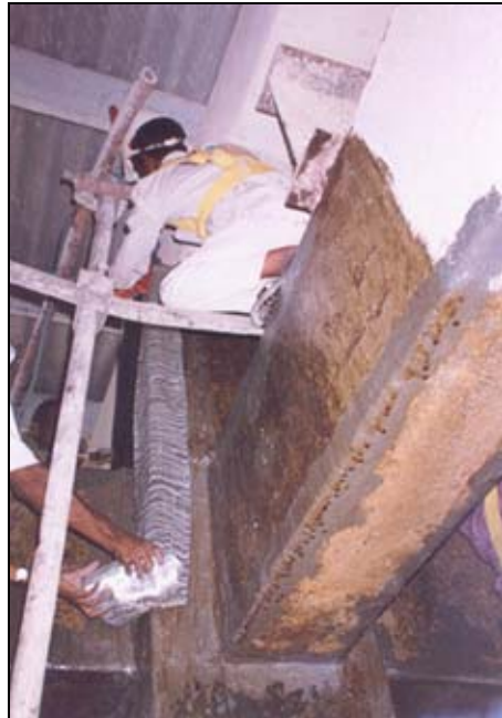
Photo 5 : Applying Saturant and E-Glass Fiber Cloth
