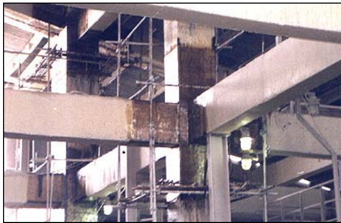
Photo 7 : Column junction wrapping in progress
