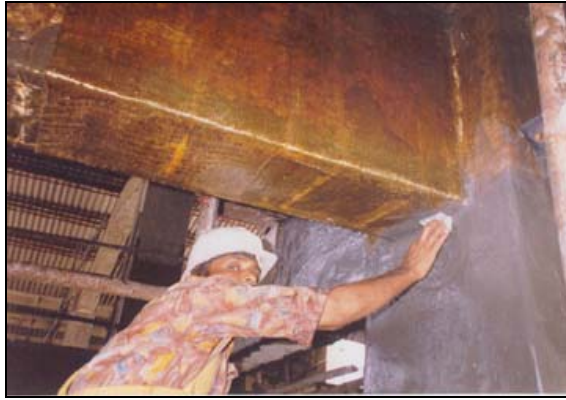
Photo 4: Putty filling and Surface preparation
