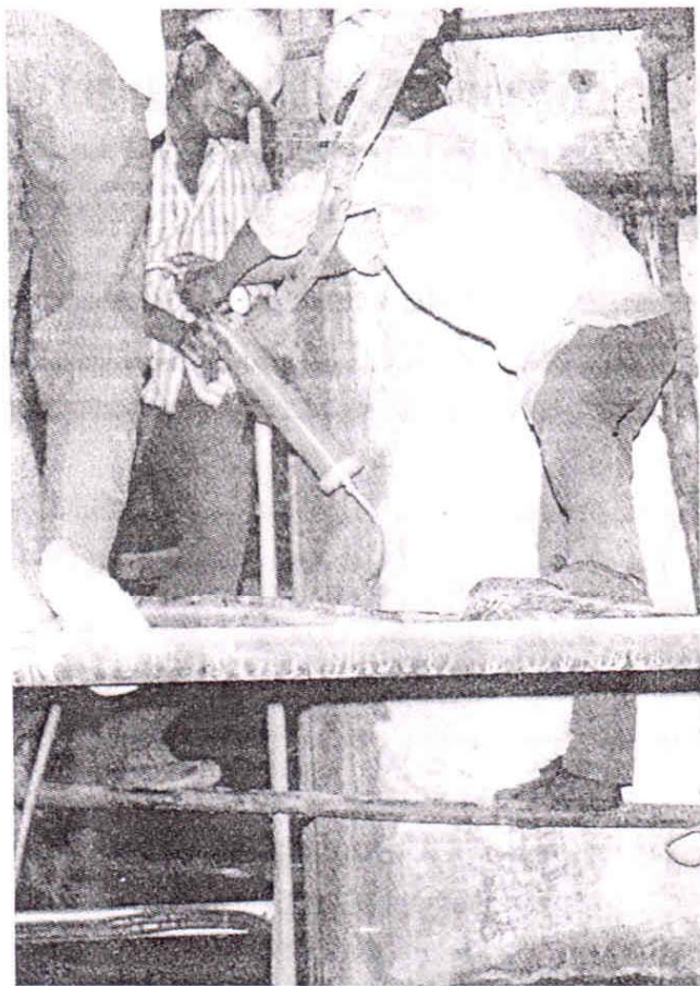
Fig 1 Strengthening of the column using epoxy resin
