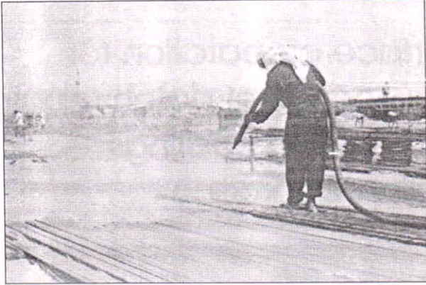
Fig 2 Sandblasting reinforcement before coating
